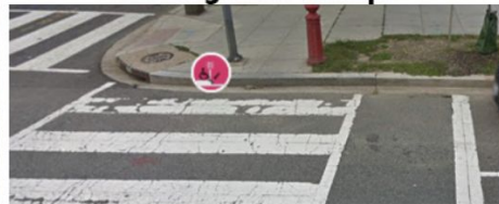
Missing Curb Ramps
